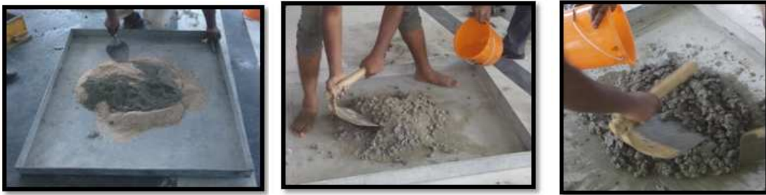
Figure 3.2: Concrete Mixing
